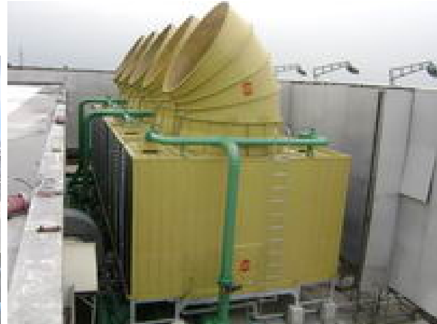
INDUCED DRAFT CROSS FLOW WITH FAN DISCHARGE HOOD
