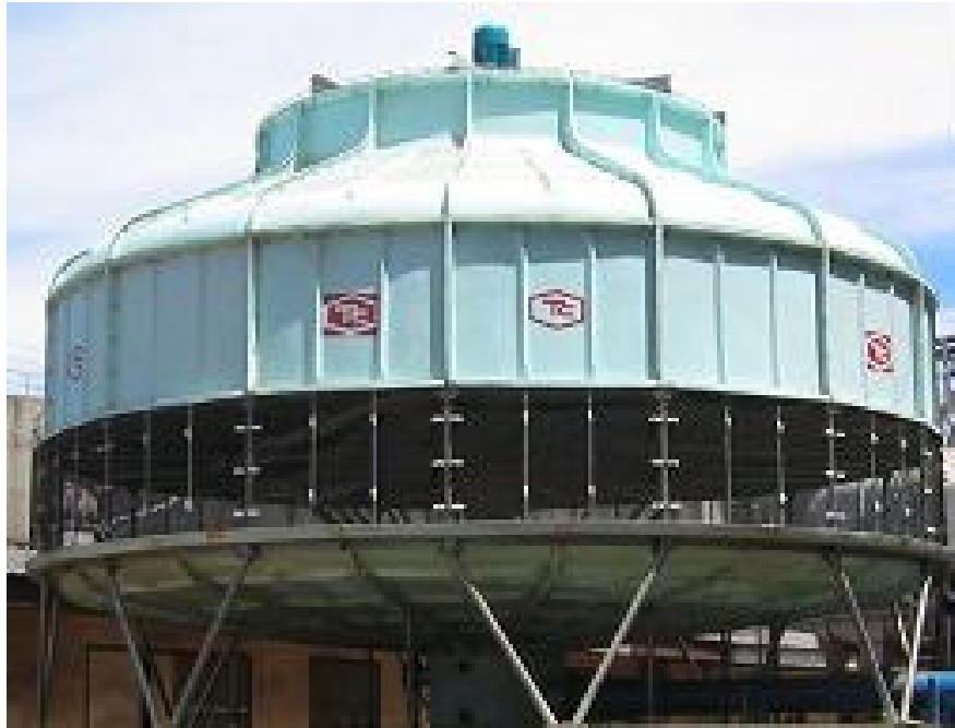
INDUCED DRAFT COUNTER FLOW
