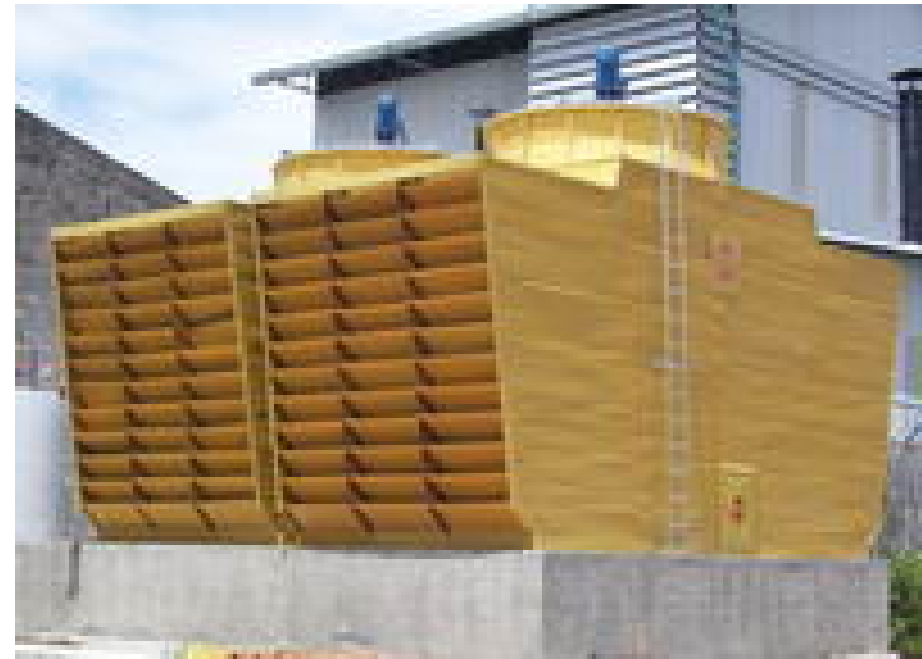
INDUCED DRAFT CROSS FLOW WITH CONCRETE SUMP
