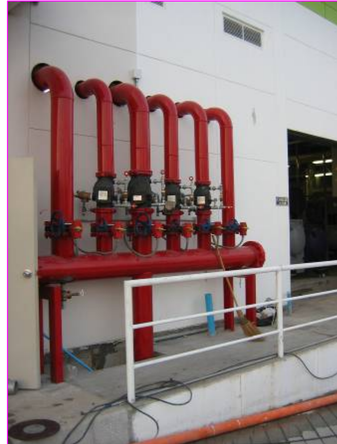
Alarm Valve Station
